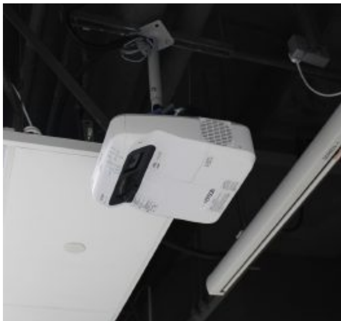
Epson ultra-short throw laser projection is employed in the Cohort Classrooms to help the spaces perform their function
