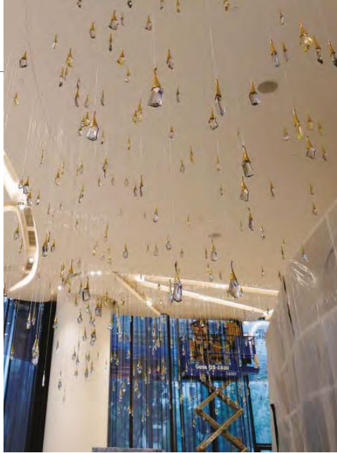
Suspended crystals in the reception area detract from the Tannoy CVS8 ceiling speakers
