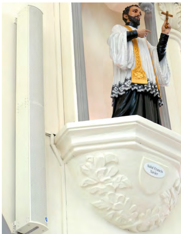
A pair of Renkus-Heinz Iconyx IC16-RD steerable column speakers provide intelligible audio throughout St Joseph's
