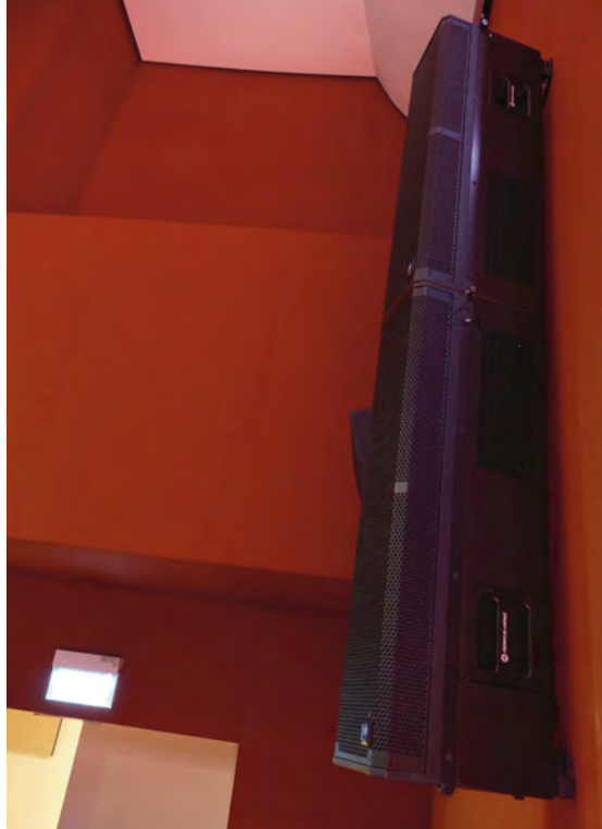
ICLive XL and ICLive LX enclosures provide full-range audio in the smaller auditorium
