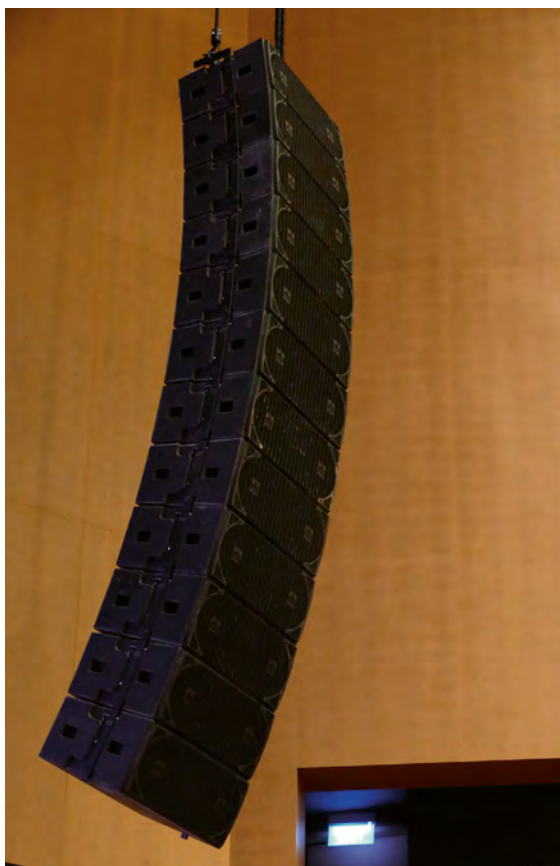
The original Renkus-Heinz STXLA 9 line array system remains in situ in the 1,400-seat auditorium
